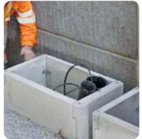
with suitable concrete slab
