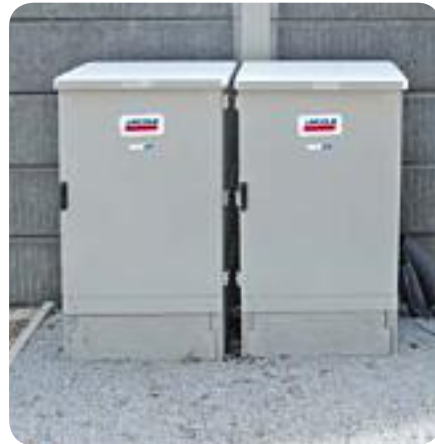
Outdoor pump cabinet 800 x 500 x 1200 mm
