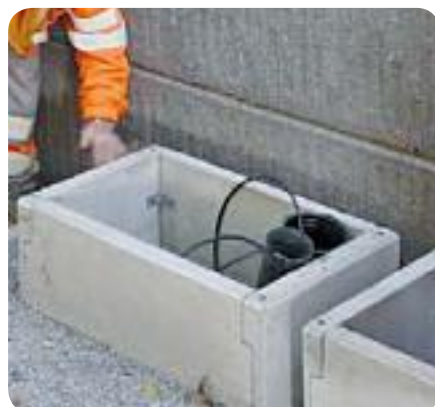
with suitable concrete slab
