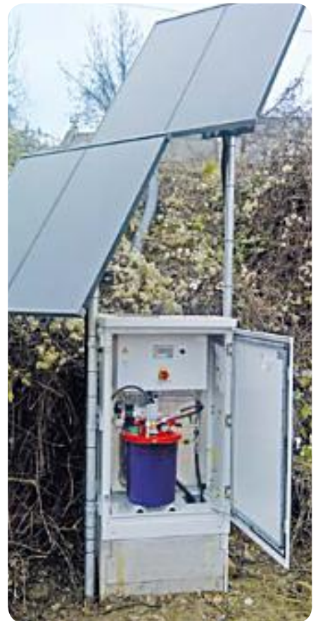
Solar unit with battery storage
