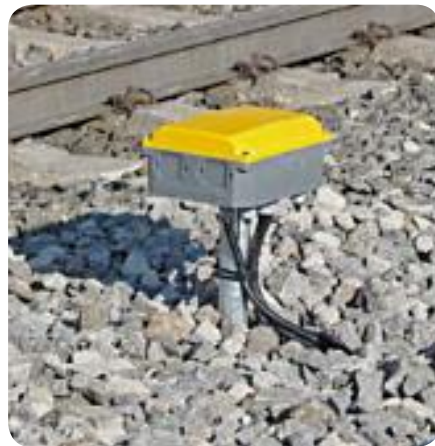
Metering device cabinet
